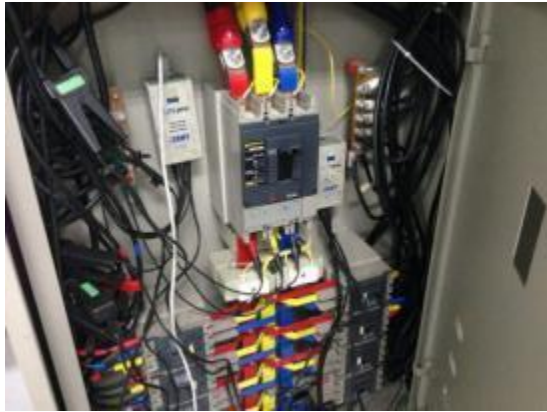
Measurement installation on Utility System By BMC
