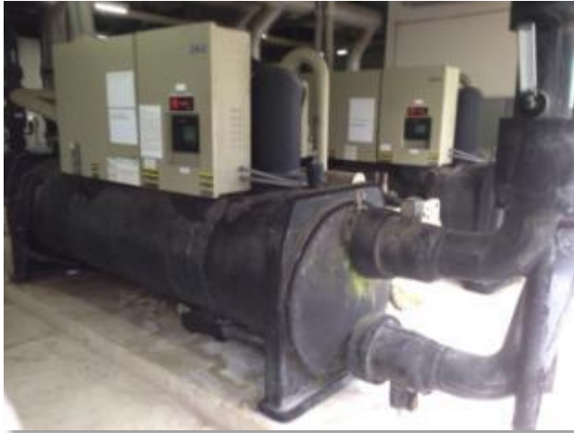
Water-Cooled chillers (350 tons x 2 units)
