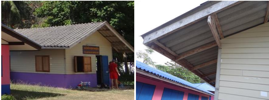
Figure 39: Rooftop sheet and structure of the public health centre
