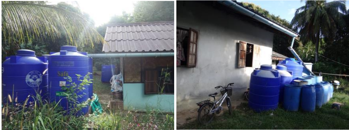
Figure 45: private storage tank collecting rainwater
