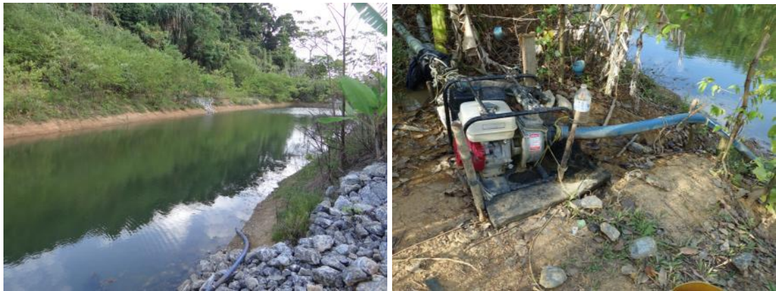
Figure 43: Large pond with water pumping
