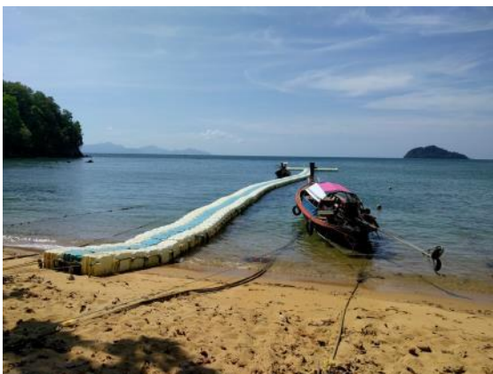
Figure 52: Floating pier at Mango Bay
