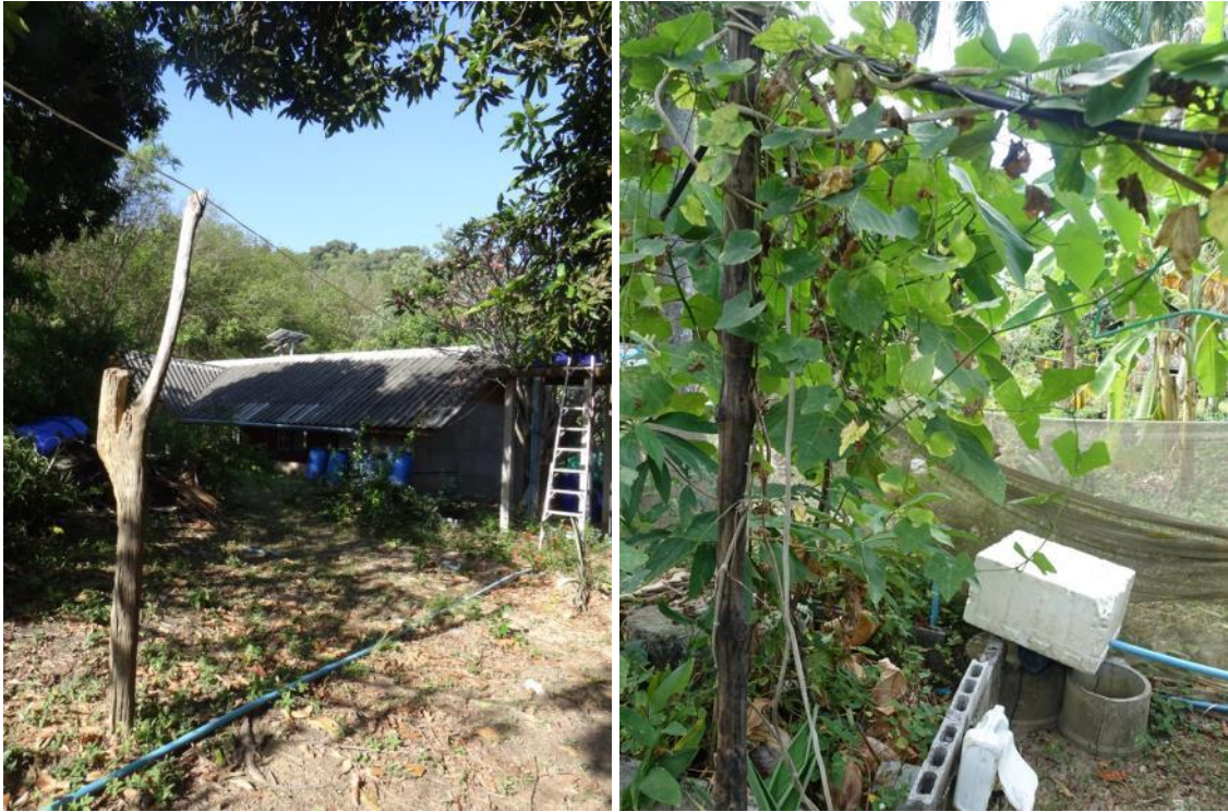
Figure 31: Wooden stick as a pole and tree connection
