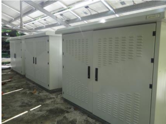
Figure 24: Battery cabinets
