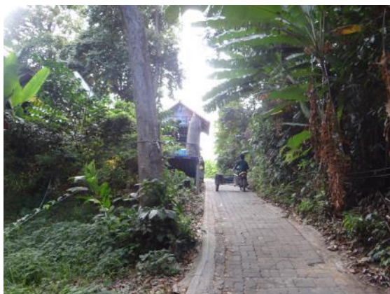
Figure 50: Typical concrete road on Koh Bulon Lae (width approx. 2 m)
