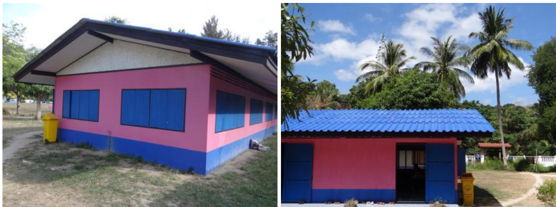
Figure 40: Rooftop sheet and structure of classroom building
