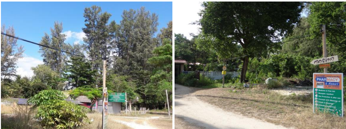
Figure 29: Grid line from school PV system to BTS2
