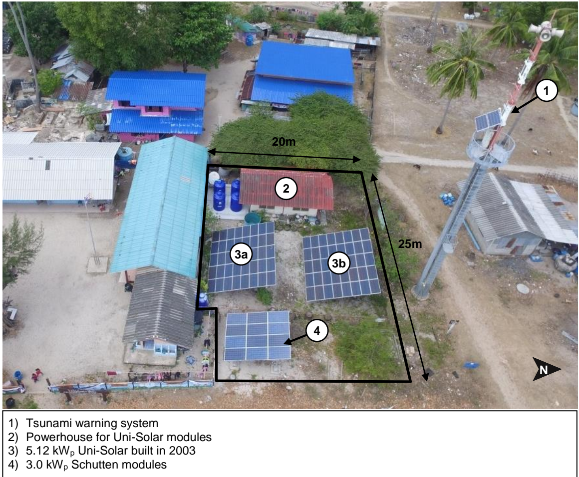
Figure 17: Overview of PV system located within school area
