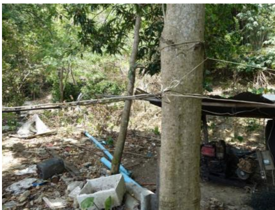
Figure 30: Grid of Generator #33
