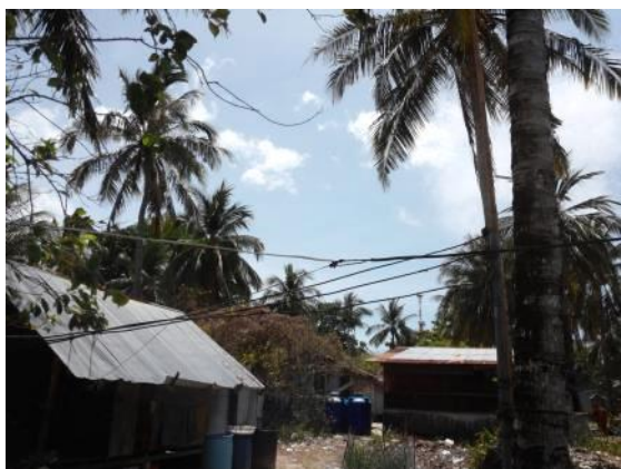
Figure 31: Grid of Generator #37
