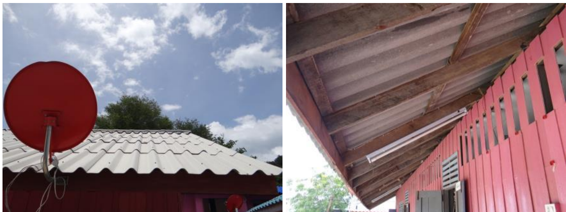
Figure 42: Roof overview and roof structure
