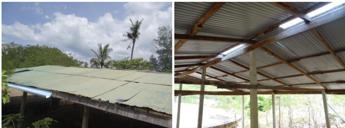
Figure 39: Structure of the roof of the building next to water storage
