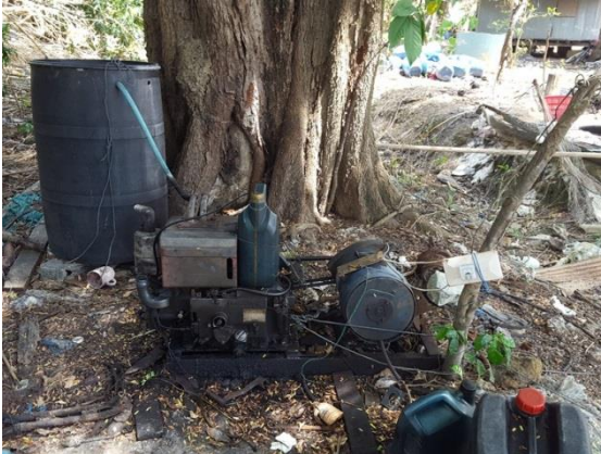
Figure 7: Generator #32a under a tree
