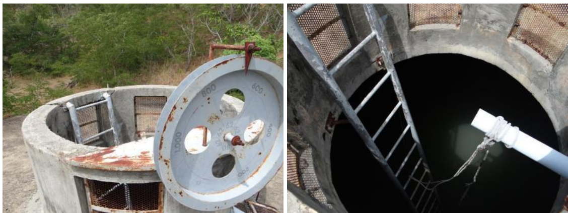
Figure 46: 1,000 m 3 water storage concrete tank
