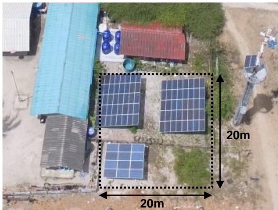
Figure 44: Existing PV area at school
