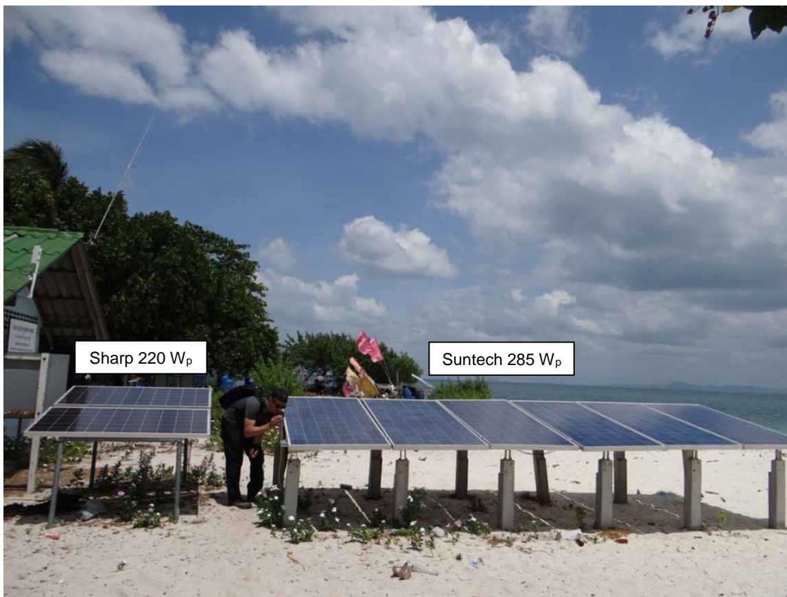
Figure 21: Two PV modules not in use [left], 1.71 kW p PV system for health centre [right]
