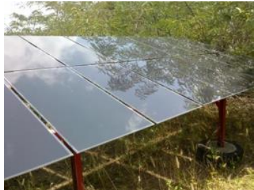
PV system @ water storage 3 kWp (for streetlights) Not working
