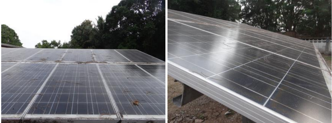
Figure 16: Dirty crystalline solar modules
