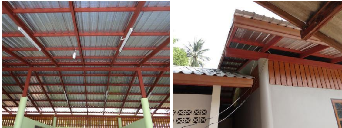
Figure 40: Roof structure and roof sheet of religion learning building (Area 6)
