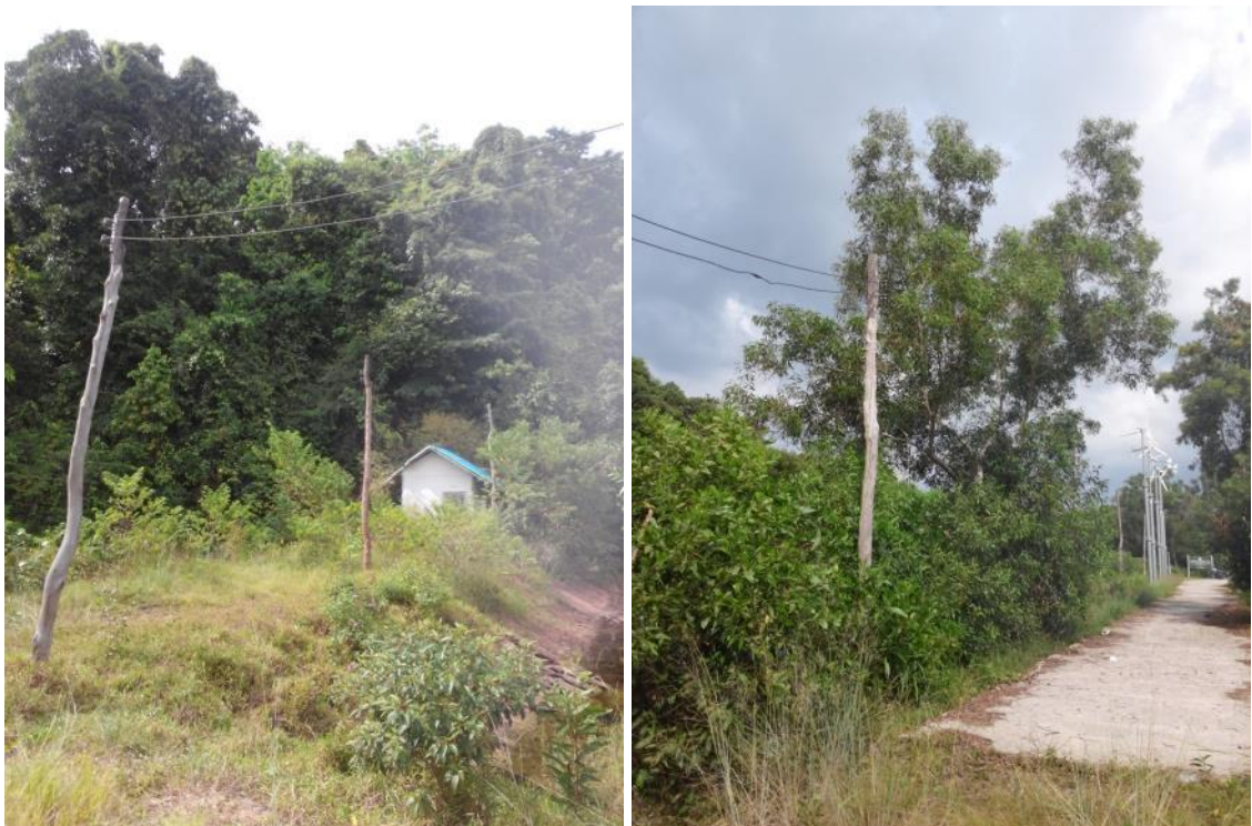
Figure 32: Wooden poles of an existing transmission line
