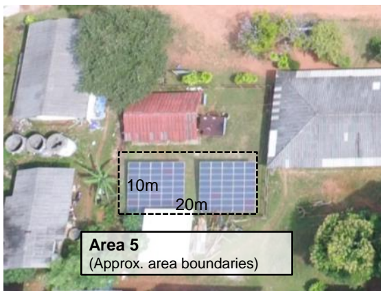
Figure 38: Existing PV area at school (Area 5)
