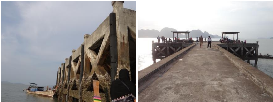
Figure 51: Koh Mak Noi pier
