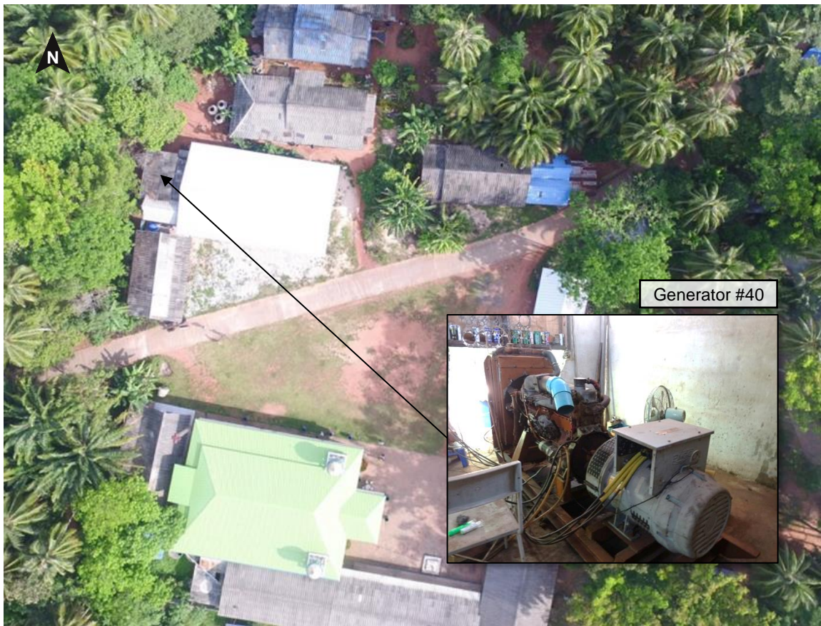
Figure 4: Powerhouse of Generator #40 within the mosque area
