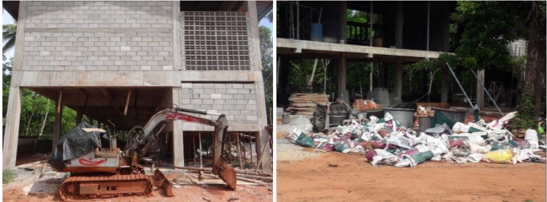
Figure 47: Excavator and manual concrete mixer
