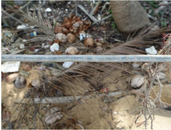
Figure 22: VAF cable in Grid of Generator #62
