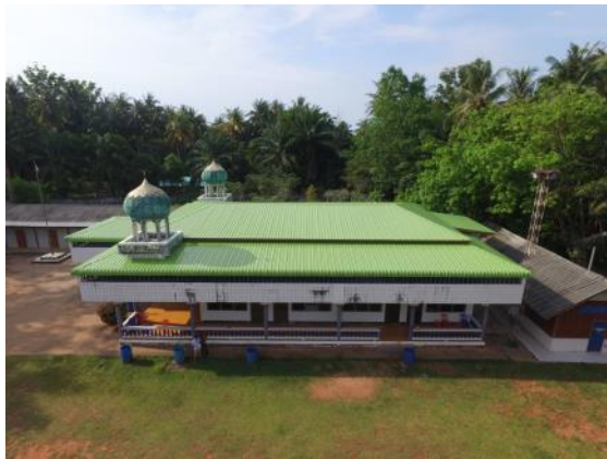
Figure 41: Mosque roof (Area 8)
