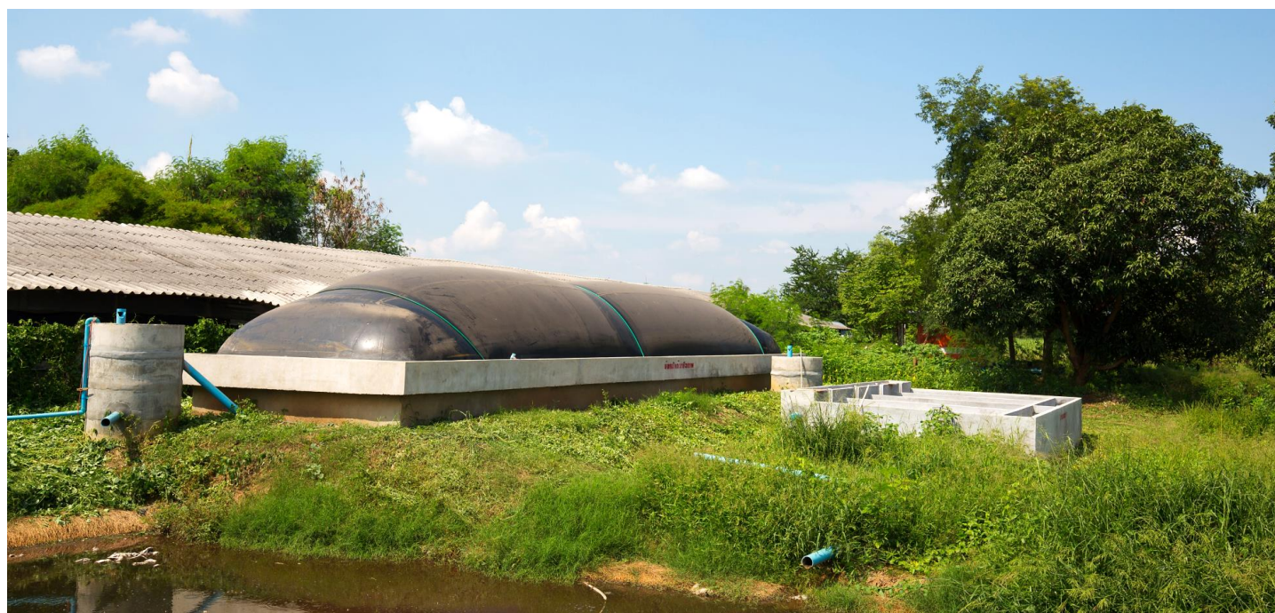
Figure 3. Biogas plant at a pig farm, Lopburi, Thailand
