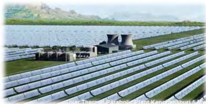
Solar Thermal Parabolic Plant Kanchannaburi 5 MW
